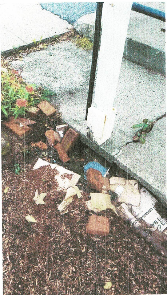
Photograph #3 – Post damage at north porch
