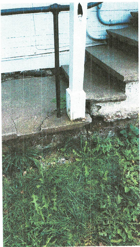
Photograph #2 – Post damage at north porch
