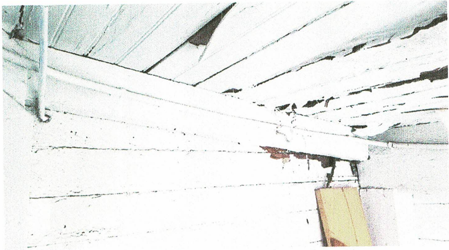
Photograph #2 – Broken rafter and damaged sheathing
