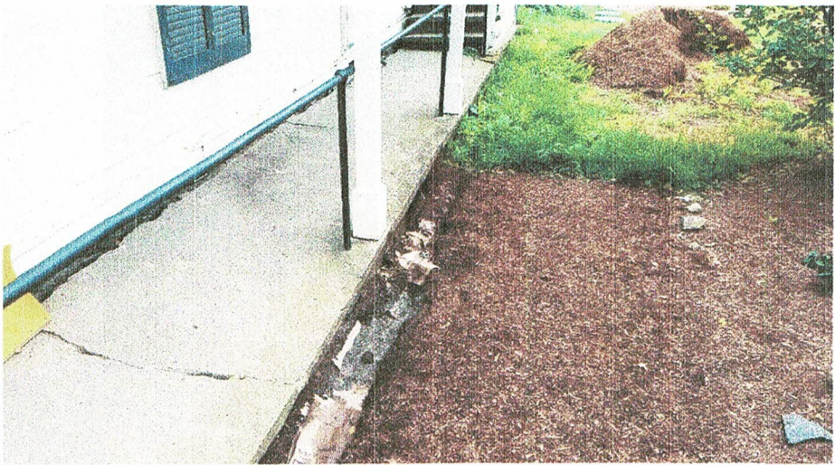
Photograph #6 – Drainage issues directed towards crawlspace access.
