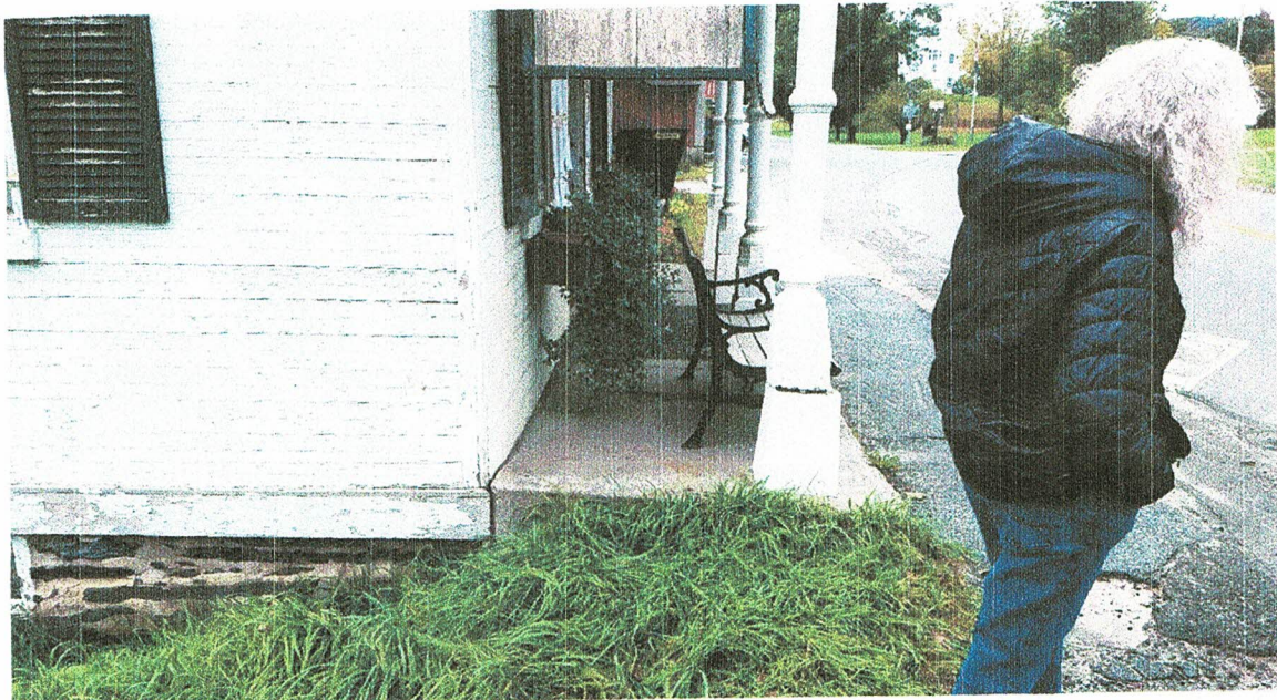
Photograph #4 – Eastern porch slope, pier movement, sill buried in concrete.
