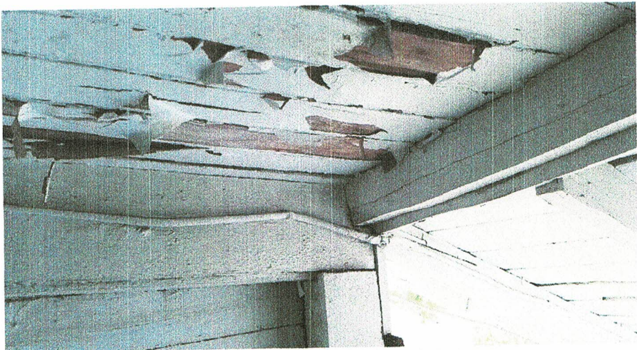
Photograph #3 – Roof sheathing damage
