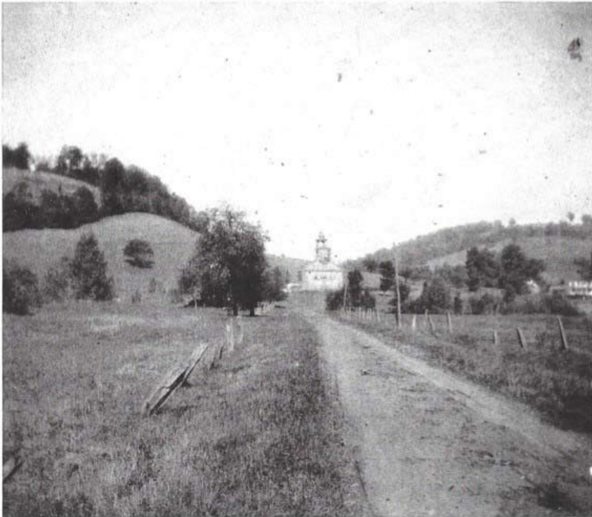
Robinson Meetinghouse, Brook Road near Sharon line, c. 1895. It was constructed in 1838.
