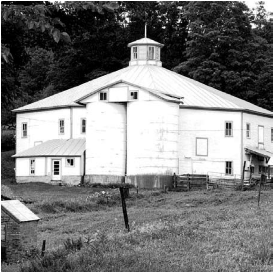
Robinson Round Barn, built 1917, 3-stories, 10-sided.
