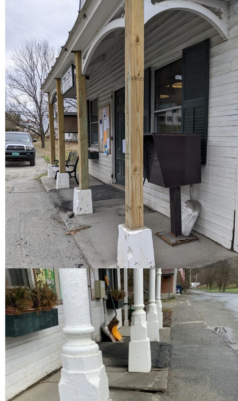
Columns 2024 (above) and 2020 (below)
